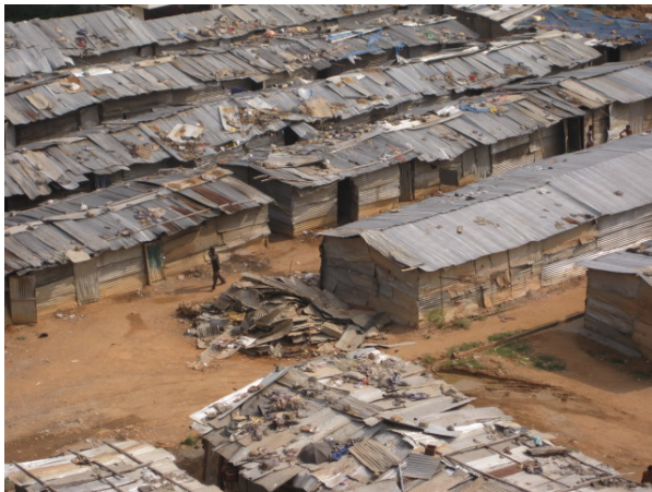
Huts near the construction site where workers live.
